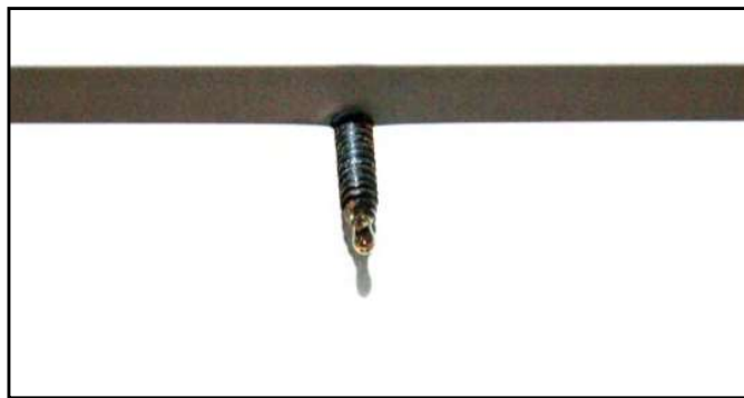
Photo 4: With 1/2” of ice in seam, melt water can run down screw threads to interior, creating life safety concerns on concrete floor below.
