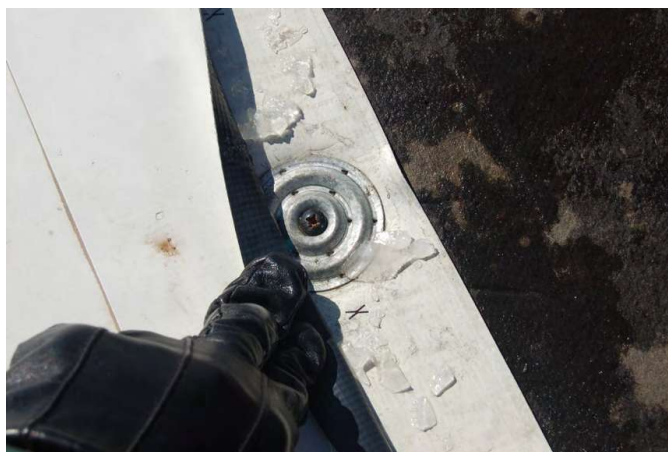
Photo 3: Note the ice should be on top of the membrane and not below.
